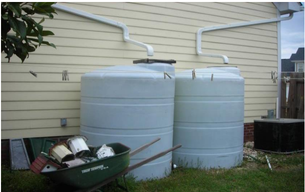
Rain Barrels with Roof Drains
